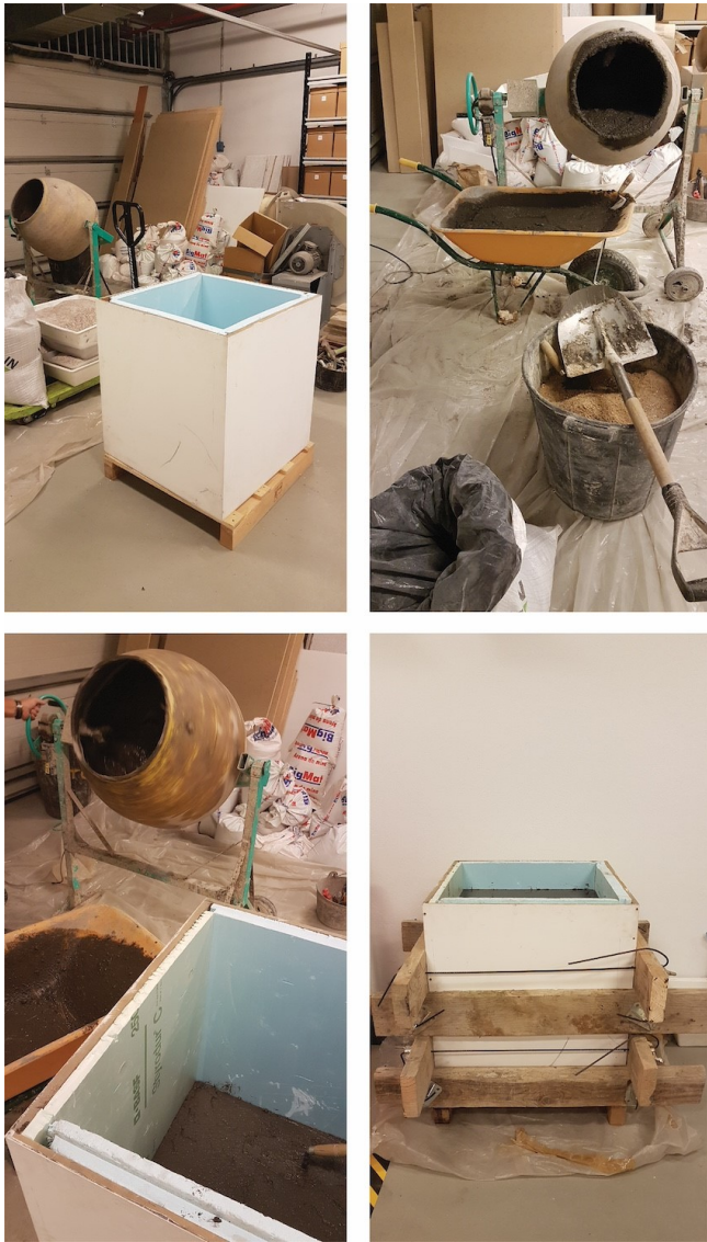
Figure A3: Construction of the Porriño granite-doped block (October 22, 2019). Once filled with the mixture, the plywood formwork was reinforced with strongly attached thick wooden boards to hold it together while the concrete block air-dried. It took the mixture almost 1 month to completely dry.
